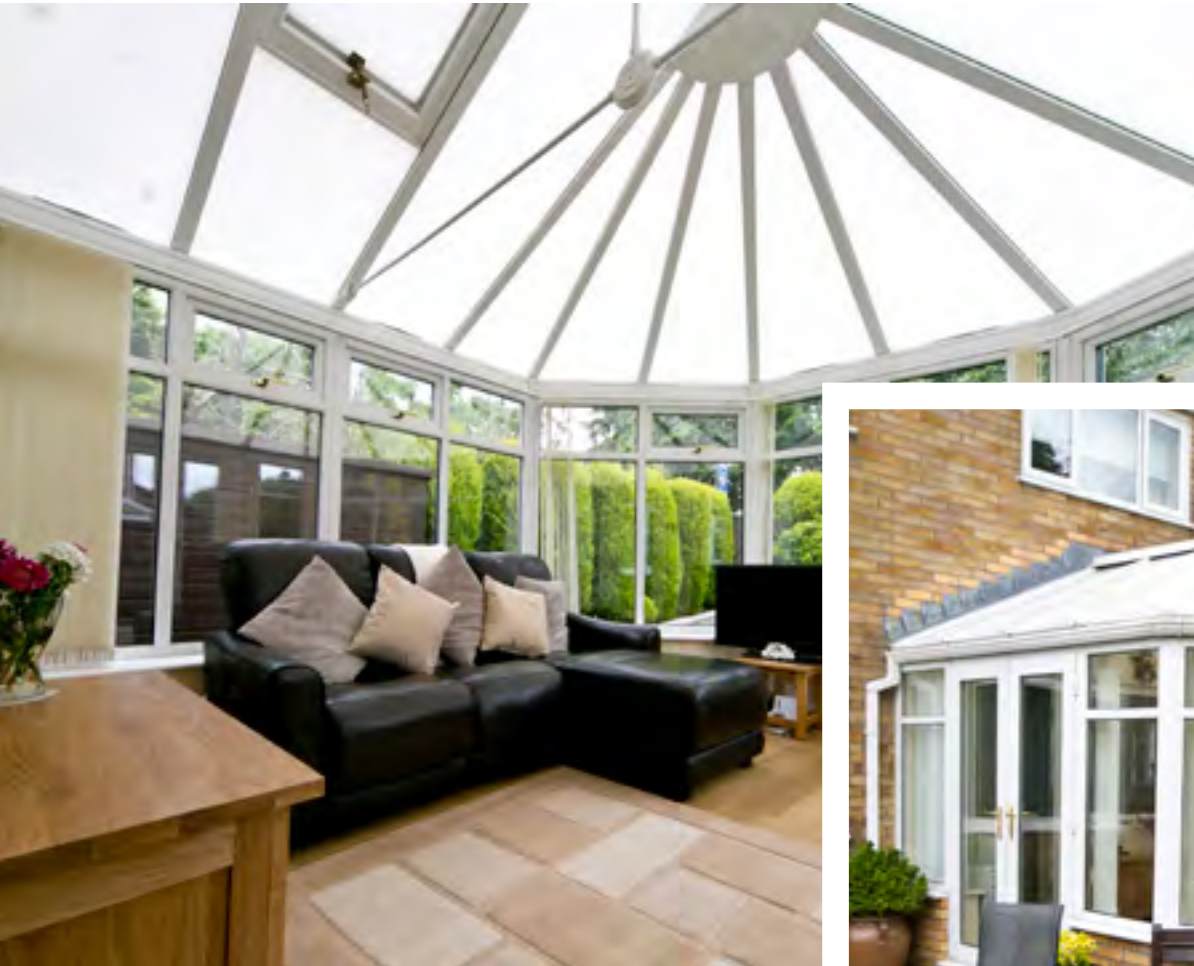
Old polycarbonate roof
