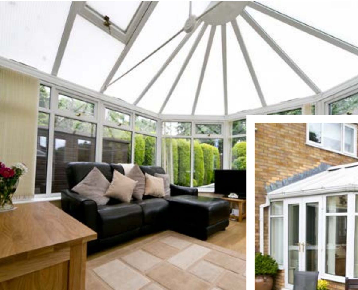
Old polycarbonate roof
